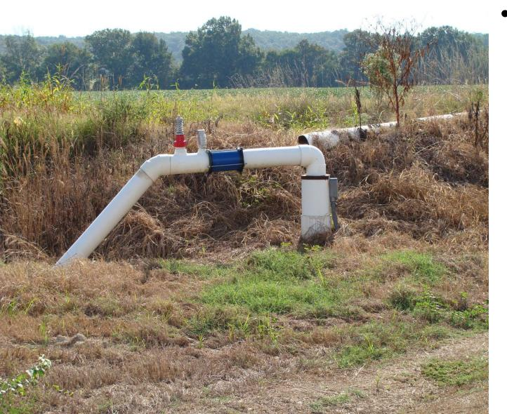
Water transfer systems were installed with risers placed in the most effective locations preventing water loss and erosion while improving irrigation efficiency.
